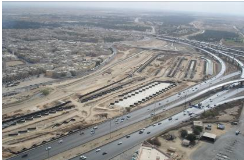
Bioremediation Facility Under construction
