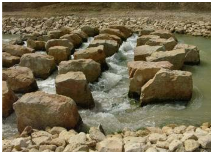
Fig. Typical Natural Stone Weir in the Dry Weather Flow Channel
